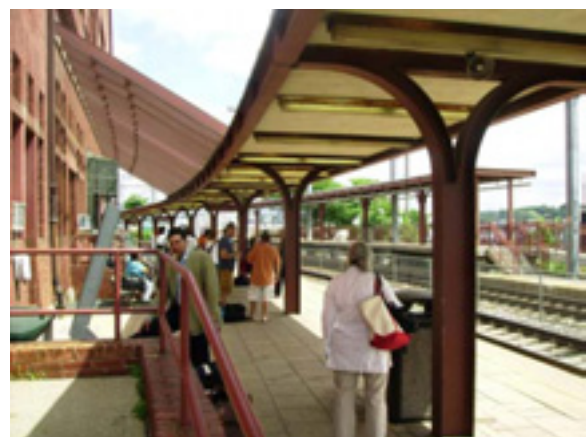
Figure 1: Union Station Rail Platforms
